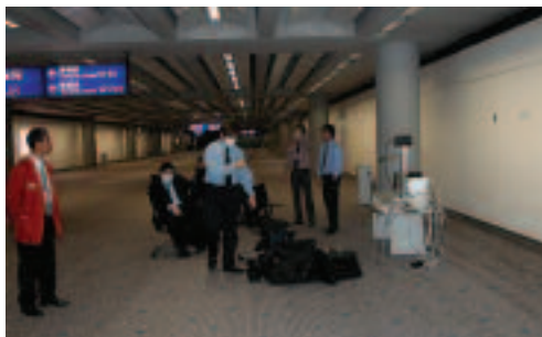
Installation of an IR system at Hong Kong airport.
